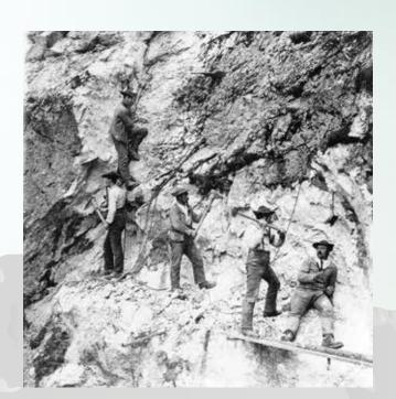
After 4 years construction time (from 1902 – 1905) the path through the gorge was finished. It took about 600 days of work, 2.500 kg explosives, 14.000 kg iron, 2.000 m water pipes, 750 m wire, 7000 kg cement and 70 kg coals for forging the iron. It cost 65.000 Mark. The ceremonial opening took place on August 15, 1905. All these men proved with their sacrificing work that it is possible to achieve something special.
